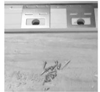
8. Install and secure the jamb with Everstrike installed to the wall frame and then add the waterstripping and latch plates.
