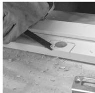
6. Place jamb leg down and install Everstrike bar and face plates face down, using the provided screws, as indicated in the figure provided below.
